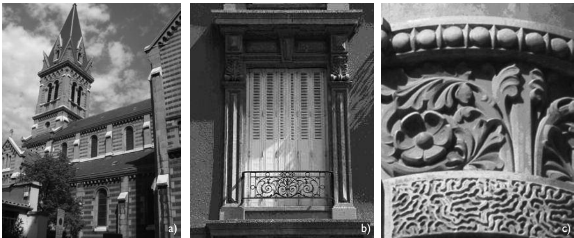
Fig. 1 Examples of natural cement applications in the French city of Grenoble: a) concrete blocks; b) window frame; c) façade ornament.
