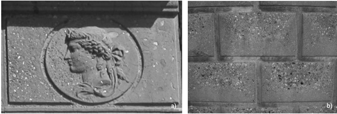
Fig. 2 Examples of erosion phenomenon observed either on sculptures (a), or on concrete blocks (b) in the city of Grenoble.
