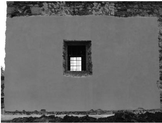
Fig. 12 Finished façade – after application of coloured lime wash.
