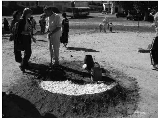
Fig. 3 Oliveirinha (Aveiro), workshop V ATP Slake the quicklime, already mixed with earth.
