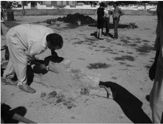
Fig. 6 Oliveirinha, workshop V ATP. Rendering adobe wall with earth-lime render.
