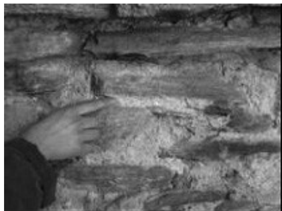
Fig. 9 An example of integration of gaps of the external plaster (above) and of the bedding mortar (below).
