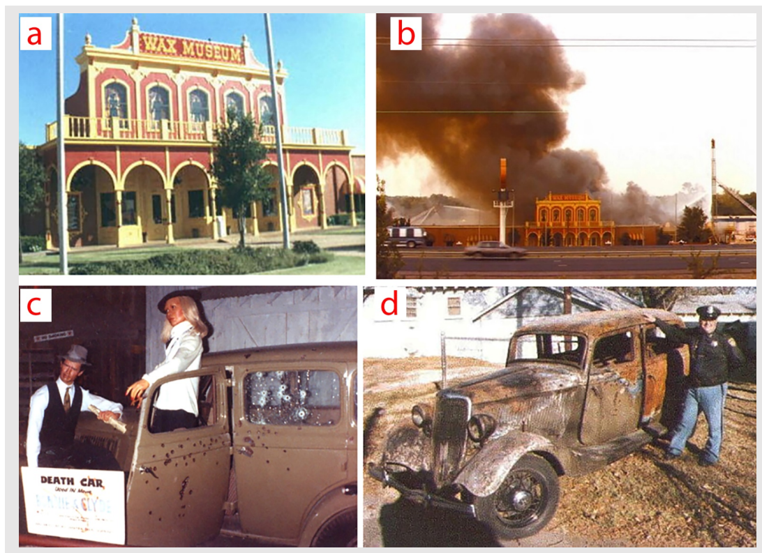
Figure 4. a) The Southwestern Historical Wax Museum in Texas; b) the same museum under the 1988 fire; c) it housed Bonnie and Clyde wax figures and the Death Car used in the homonymous; d) the fire destroyed the wax figures completely, and caused severe damage to the car. Original photographs from Ballinger, F.R. 'Bonnie and Clyde wax display-the Southwestern Historical Wax Museum' (n.d.), in Bonnie & Clyde's Hideout , http://texashideout.tripod.com/wax.html (accessed 2019-12-01)
